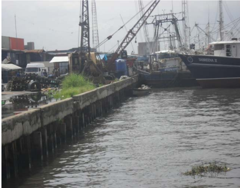
Fig. 12. OILY WATER CAPTURED AT KLT I
