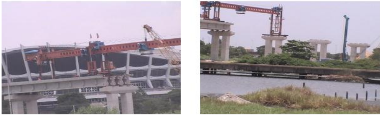
Figure 22: on-going Monorail Terminal Construction
